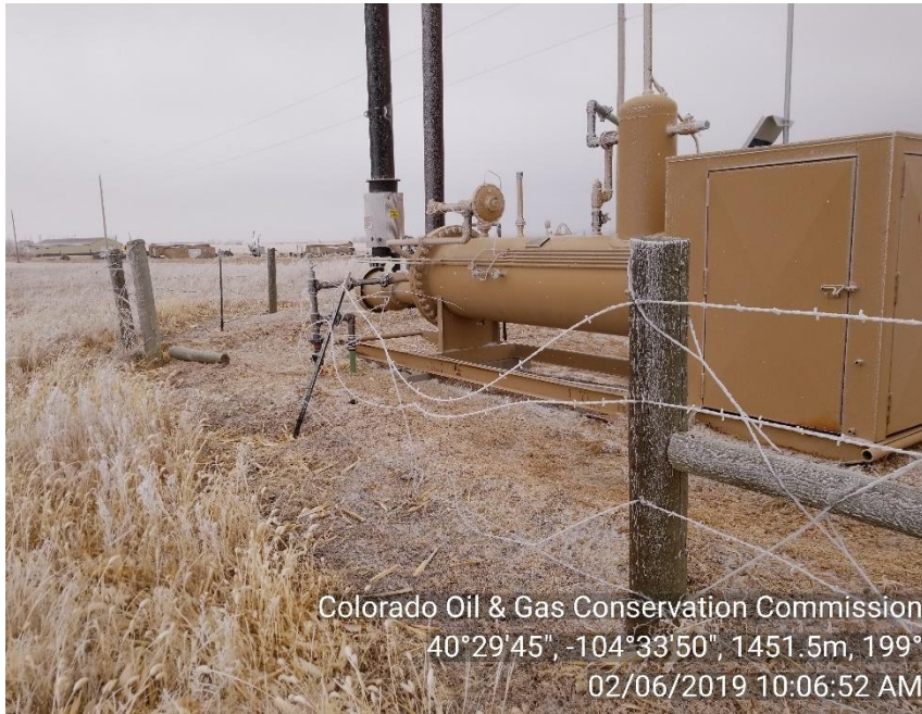
Photo 3: Fence around separator in disrepair.
