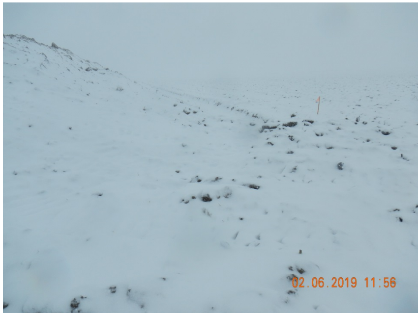
Photo 3. Photo taken from northeastern perimeter of the location, facing West. Photo illustrates the ditch and berm BMP that has been installed around the perimeter of the location has been tracked through by equipment and opens to adjacent field with no stormwater BMP or stabilized outlet.
