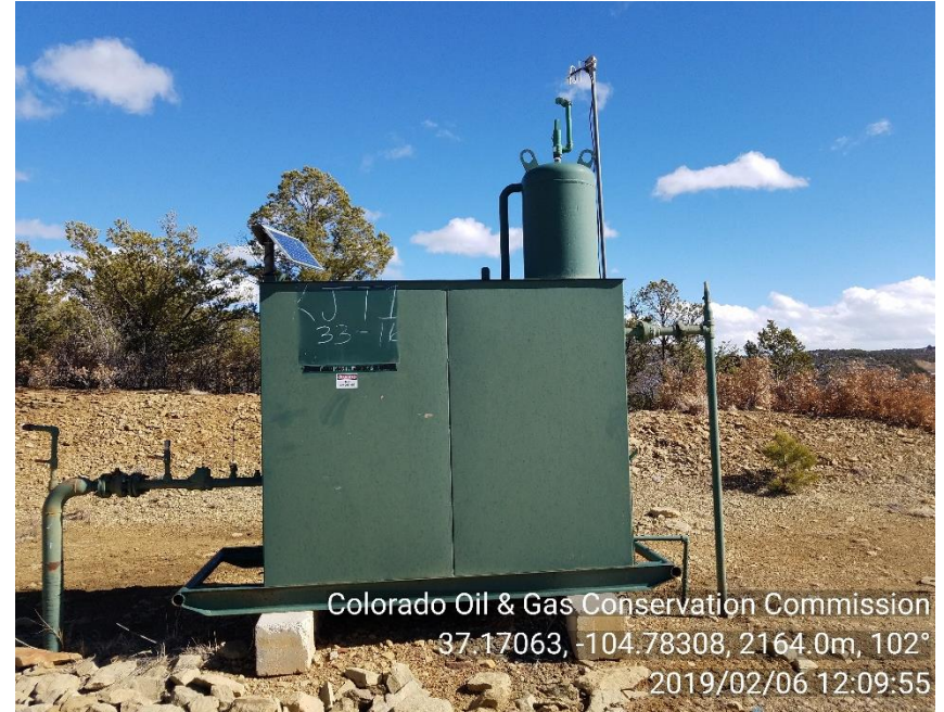
PHOTO 2: WELL SIGN/METER HOUSE/ SIGN NOT POSTED/ NO EMERGENCY CONTACT NUMBER POSTED
