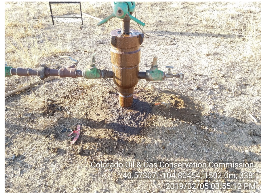
Photo #4 Law 1-17 Wellsite Stained soil & fluids on wellhead
