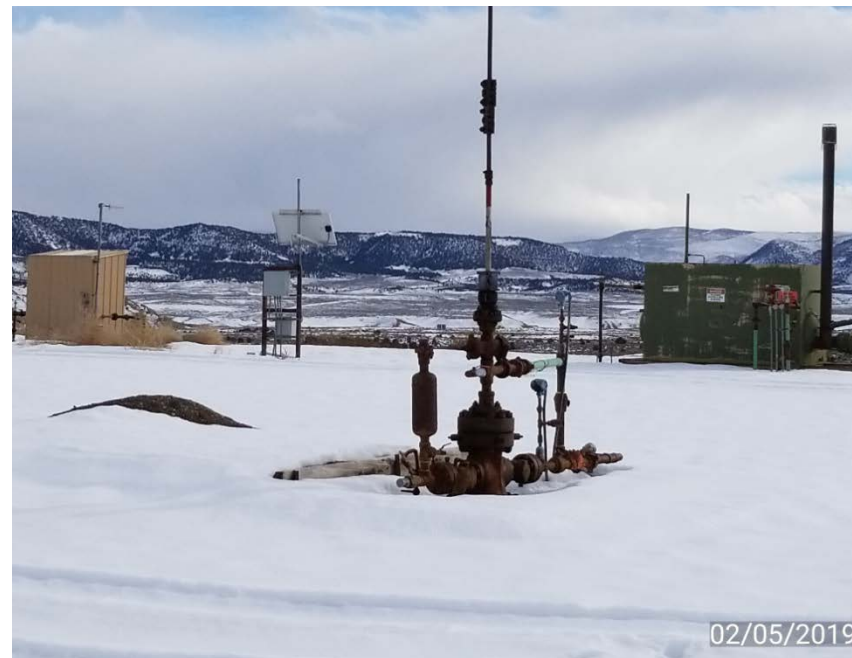
Photo 2. Well head, separator, and gas meter building.
