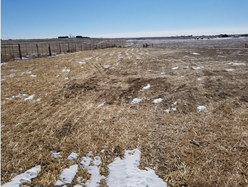
Photo 1. Photo taken from the access road of CR , facing South. Appears the Operator has performed final reclamation activities, with the evidence of drilling rows and straw crimped mulch.
