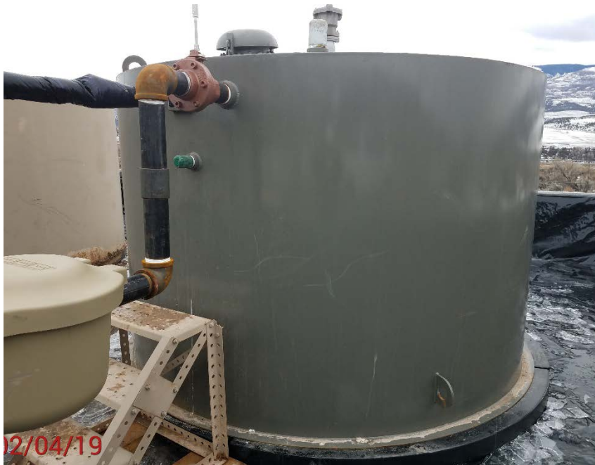
Location Photo #5, Missing tank labels.
