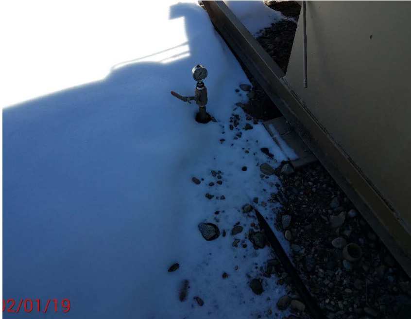
Location Photo #5, unmarked flow line riser.
