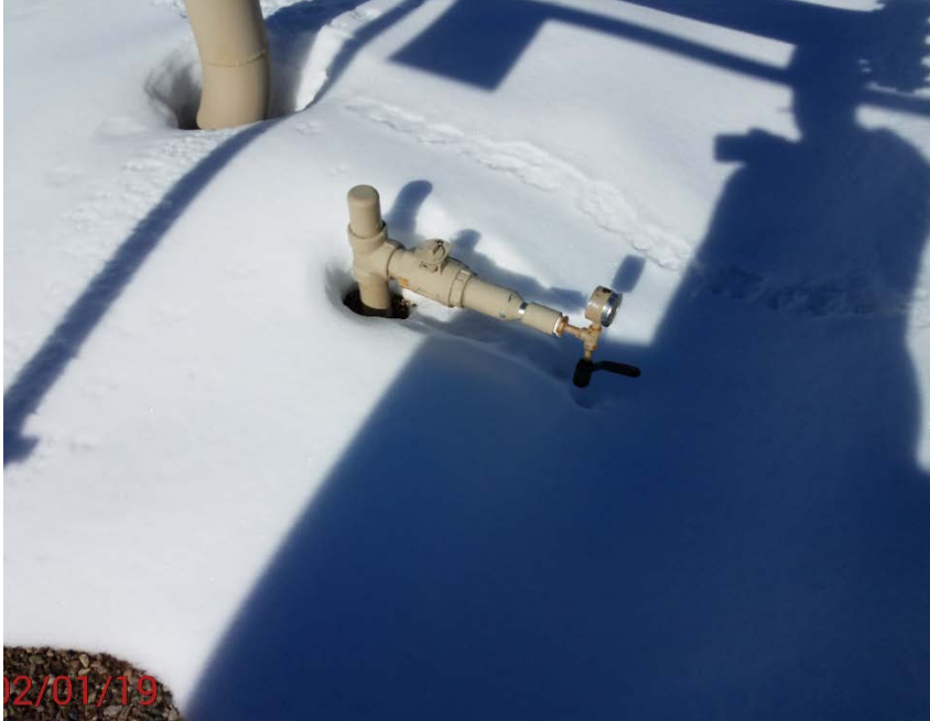
Location Photo #7, unmarked flow line riser.
