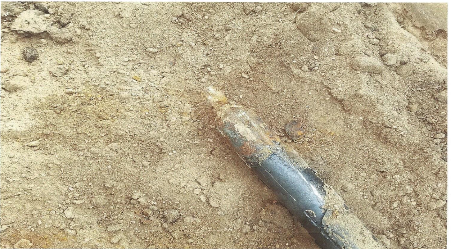
South End of Flowline Discovered Previously Capped
