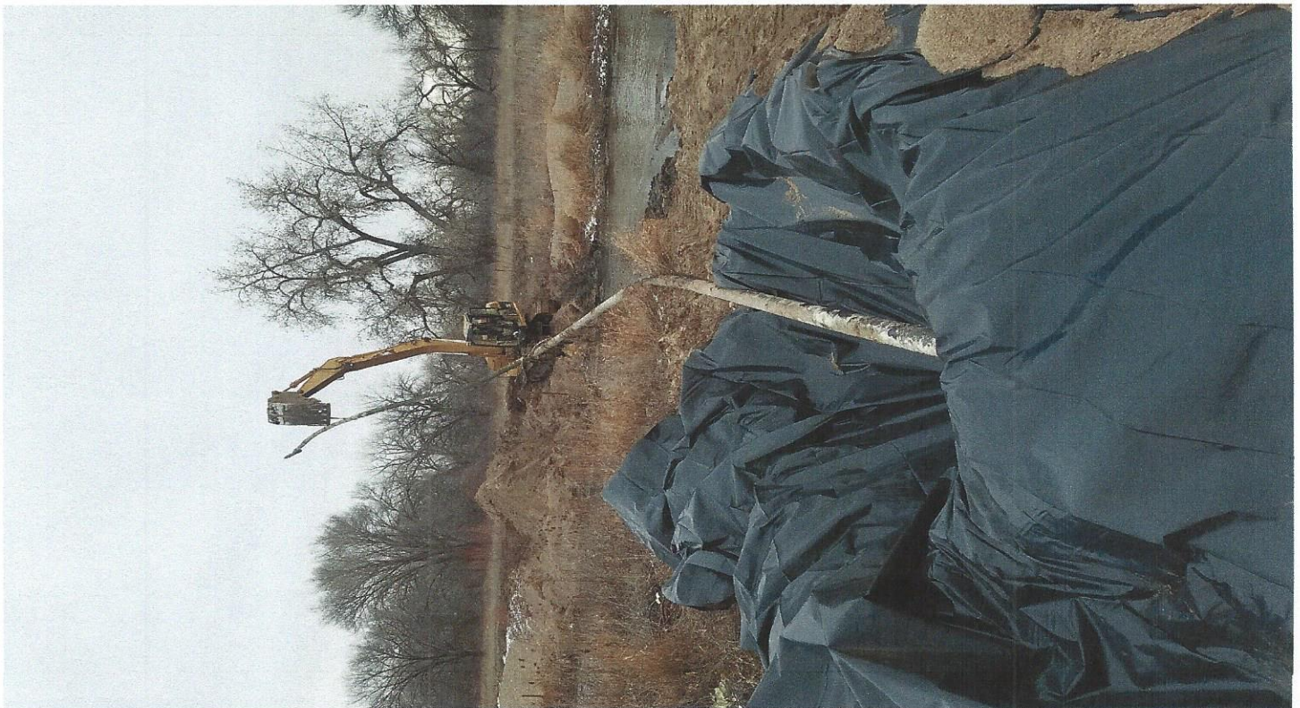
South End of Flowline raised to adequate height in order to purge line of fluids
