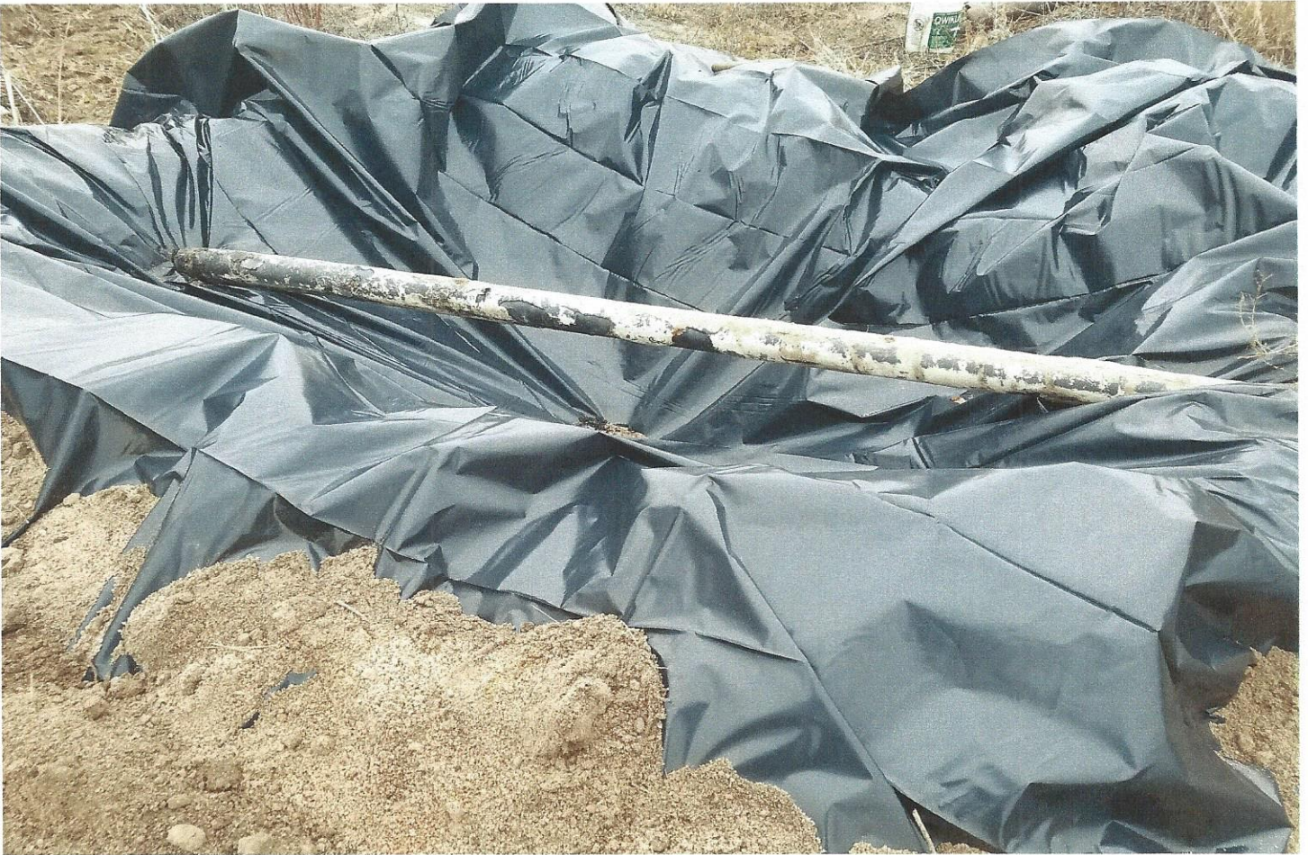
South End of Flowline raised to adequate height in order to purge line of fluids
