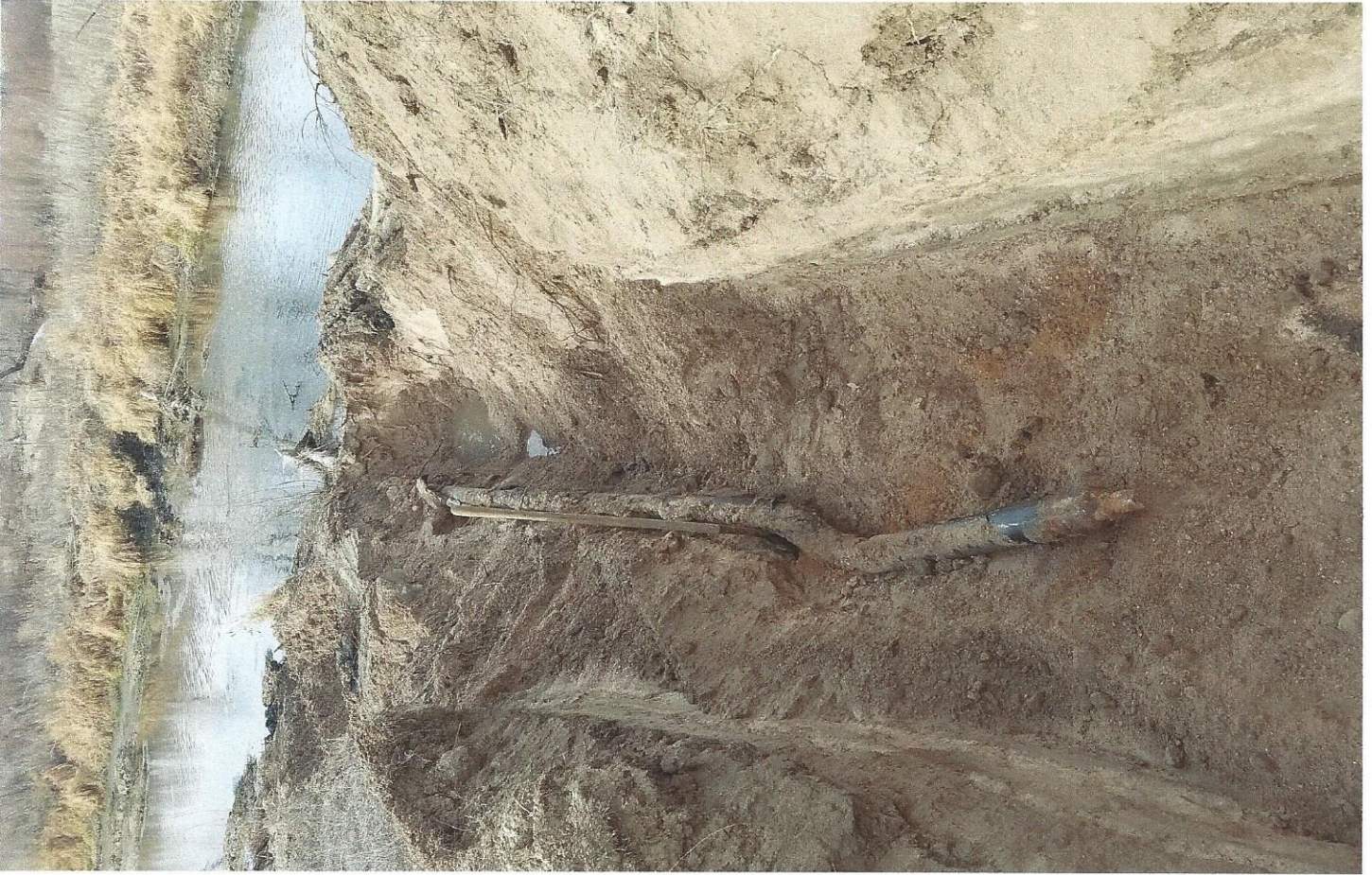
South End of Flowline Discovered Previously Capped
