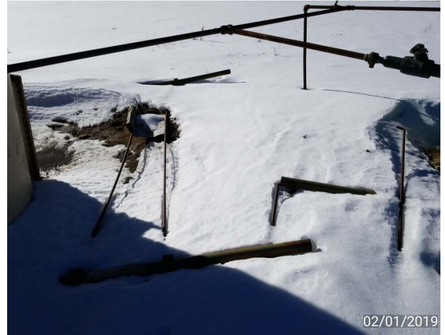
Photo 2. Well head sign lying on ground next to tank and missing nearest public road "CDR 27".
