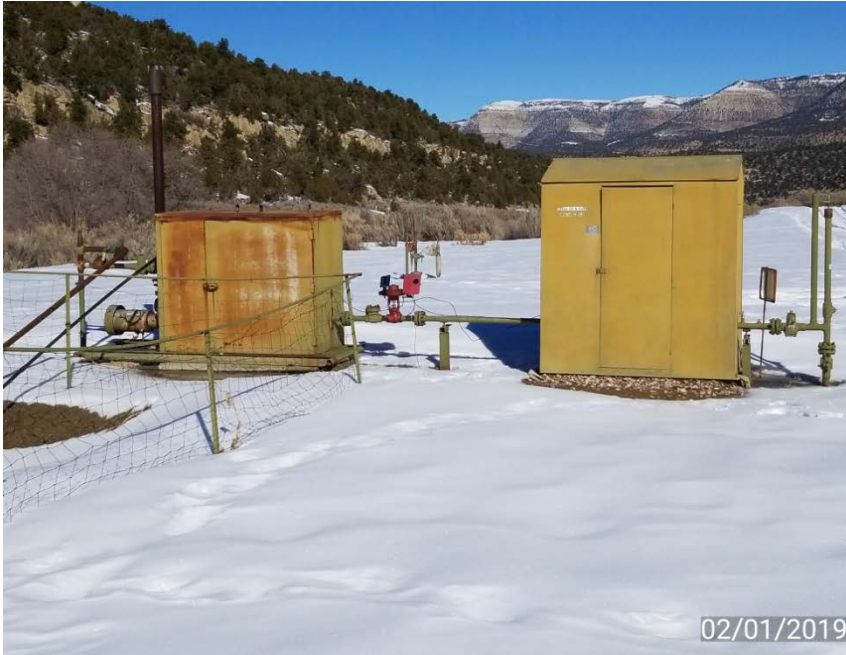
Photo 1. Location looking north.
