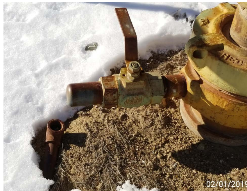
Photo 2. Riser next to well head not capped or LOTO.
