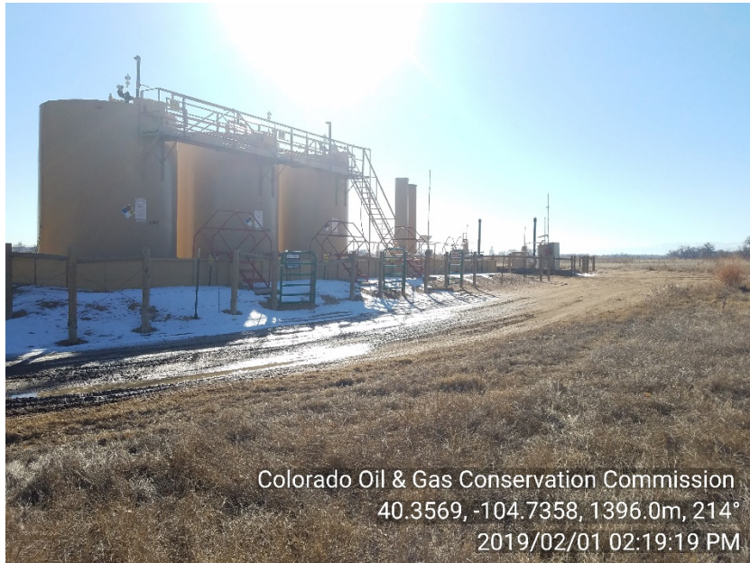
Photo #1 Schank J 35-7, 35-08, 35-17, 35-22 Battery site
