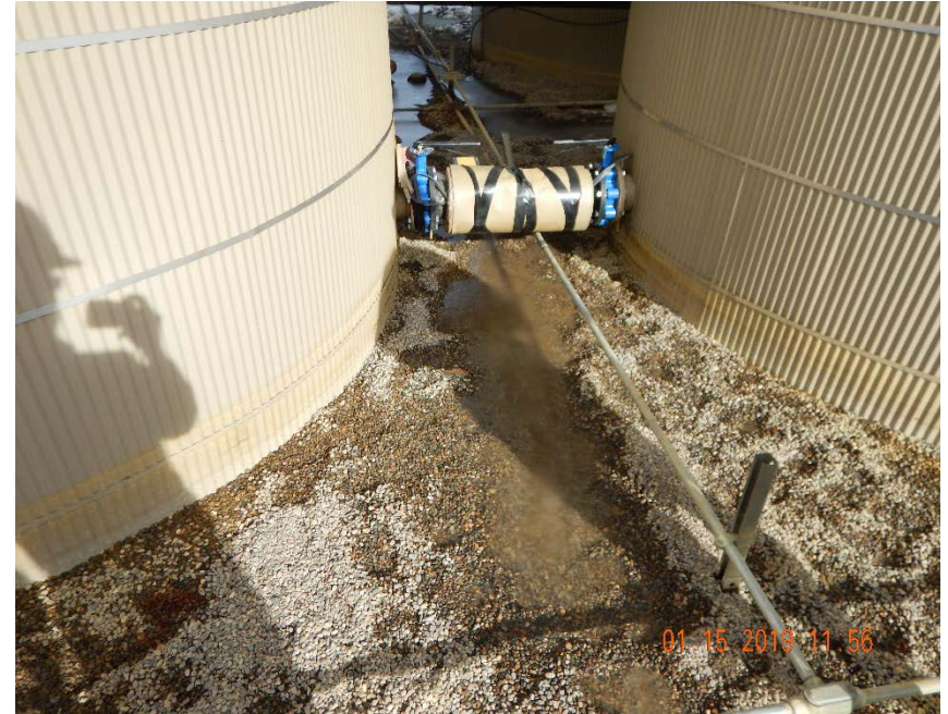
Photo #6 – View of tank leveling pipe that was the source of fluids released by Spill/Release ID #460723 from south side of tank battery.
