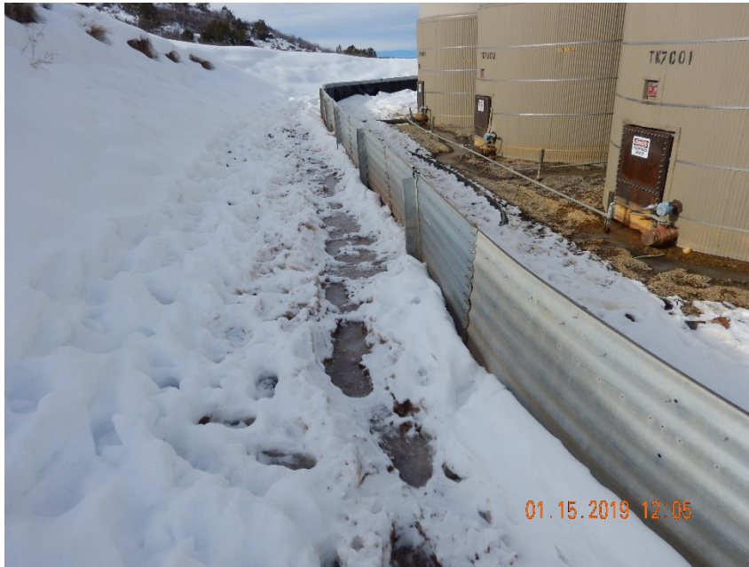
Photo #7 – View of areas inside and outside of tank battery SPCC from east side. Operator indicated that fluids released during Spill/Release ID #460723 had impacted soil outside of SPCC.
