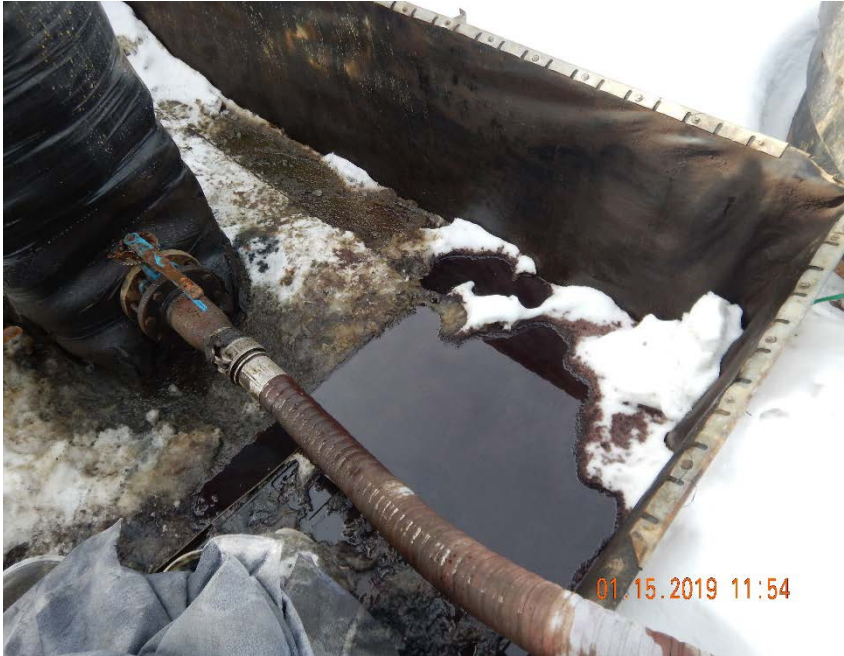
Photo #5 – Free product inside of SW tank battery truck loadout SPCC. Refer to R. Murray’s inspection (doc #693200212) for corrective action.
