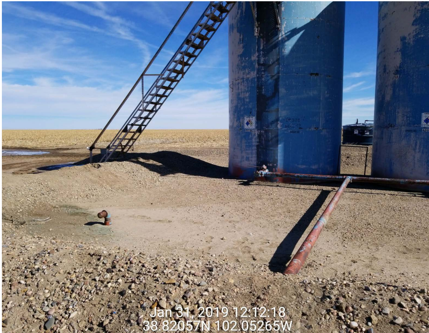
Unmarked pipeline risers
