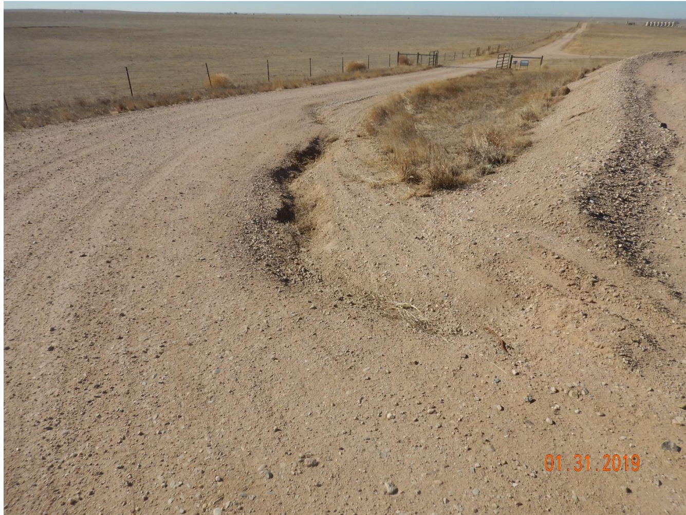
Photo 11: Photo taken from the access road on the south end of the location, facing southwest. Photo shows erosion degradation along access road due to stormwater runoff.
