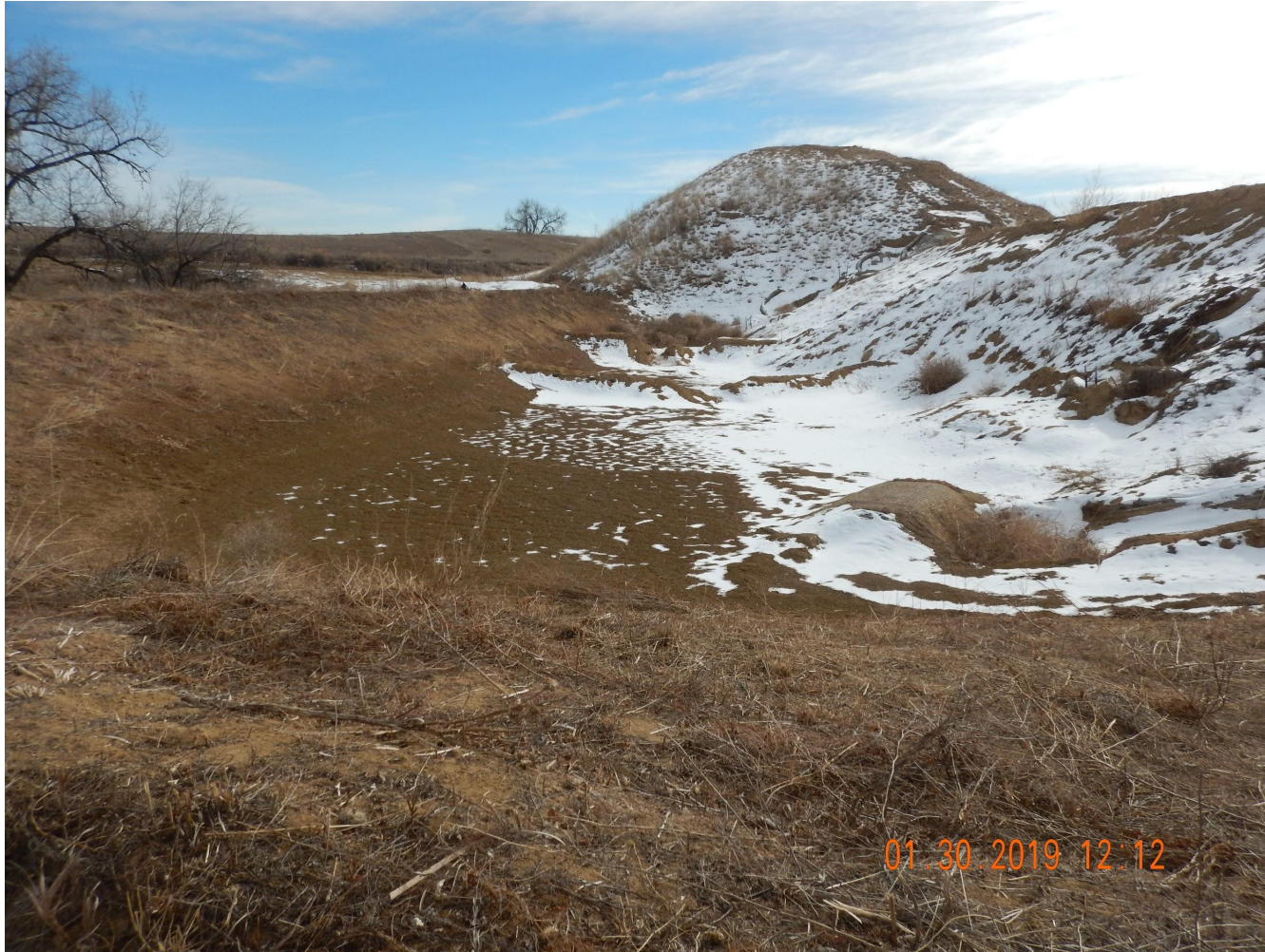
Photo 11. Photo taken from the northeast perimeter of location, facing South. Photo illustrates the sediment basin. Maintenance is needed, as gully erosion was observed along portions of the inlet- see following photo.
