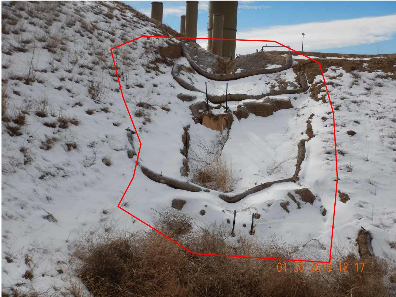
Photo 12. Photo taken from the southern inlet for the sediment basin, facing West. Photo illustrates maintenance is needed, as gully erosion was observed. Operator has failed to maintain BMPs per Rule 1002.f.
