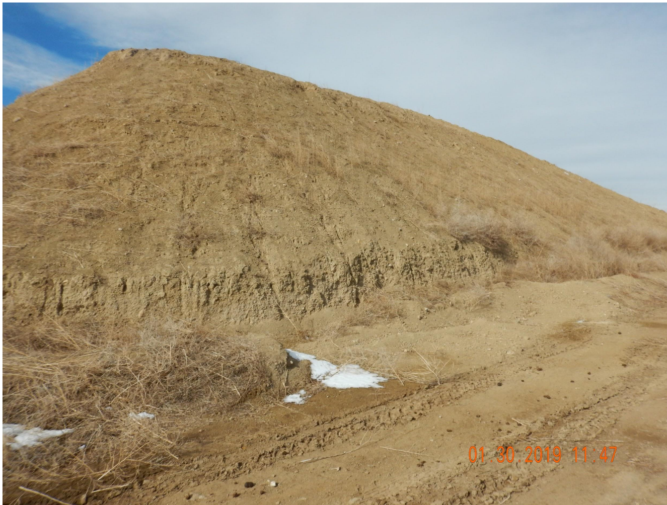
Photo 4. Photo taken from the southeast perimeter of location, facing Northwest. Photo illustrates rill erosion along the southern slope of the stockpile and unmanaged weeds. Rill erosion was observed throughout most of the location. Operator has failed to adequately stabilize stockpiles and fill slopes to minimize erosion and site degradation per Rule 1002.f.
