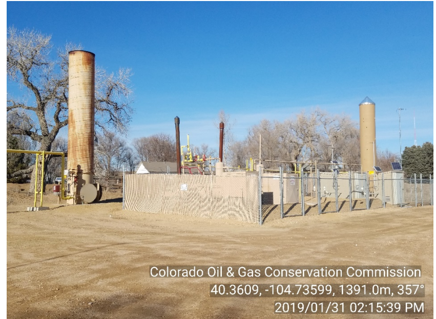
Photo #2 Schank J 35-1, 35-27, 36-31 Battery site – Separators, ECDs, Gas meters
