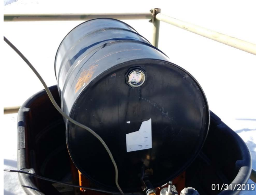
Photo 2. Container next to well head without labels.
