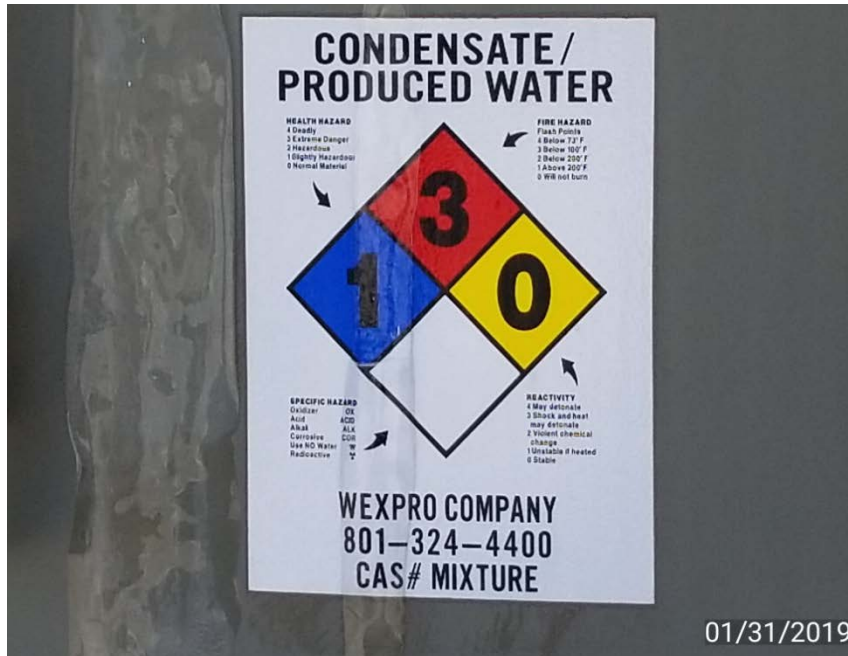
Photo 3. Tank label missing current operator, phone number, and capacity.
