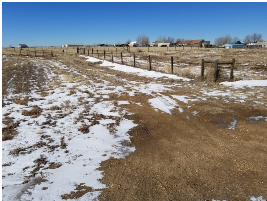
Photo 1. Photo taken from the access road looking into the location, facing West. Operator has performed reclamation activities. However, the location lacks uniform perennial vegetation and are covered in weedy, annual vegetation which includes but not limited to cheatgrass and kochia. The access road remains.
