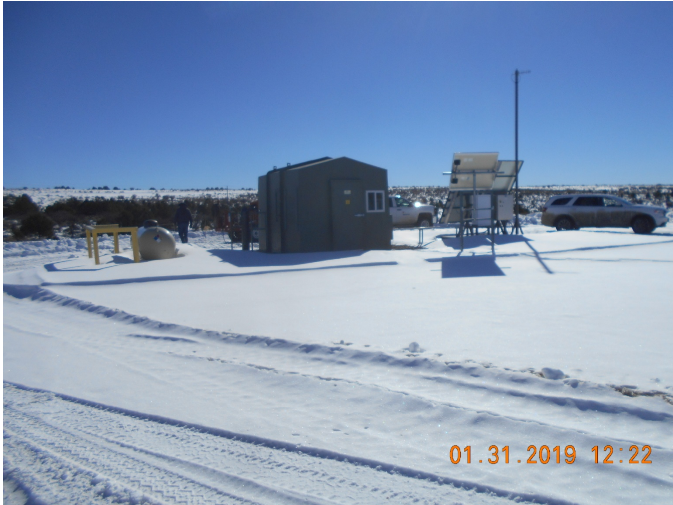
Injection wellhead housing
