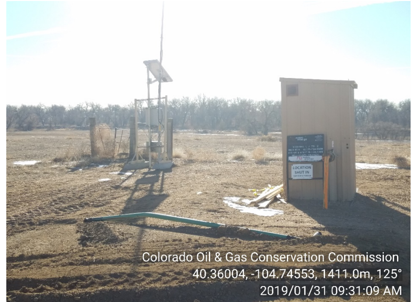
Photo #3 Schank #1, J 35-2 Battery site Abandoned Unused Equipment Gas meter run, line pipe, automation controls
