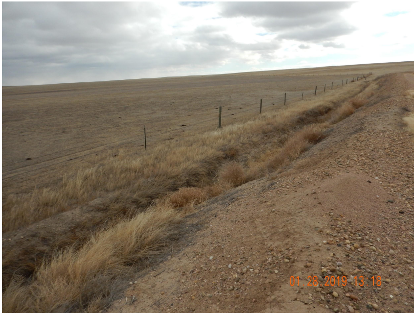
Photo 3. Photo taken from the eastern well pad, facing South. Photo illustrates unmanaged weeds along the fill slope. Operator shall control weeds and weed debris per Rule 603.f.
