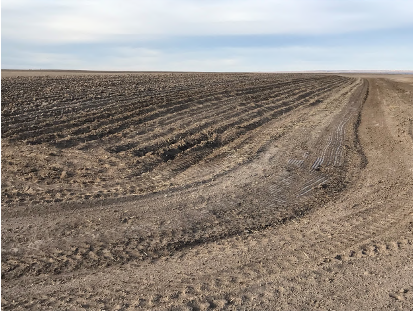
South west corner of pad – looking north/northwest at topsoil stockpile. Topsoil pile tracked and ditch BMP installed
