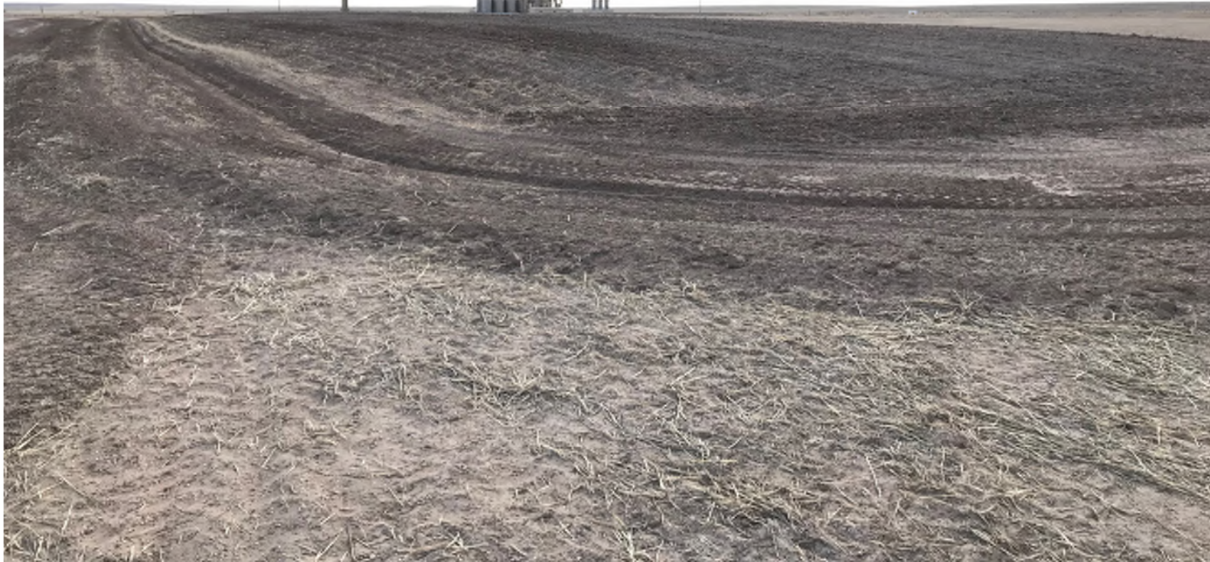
North west corner of pad – looking south/southwest at topsoil stockpile. Topsoil pile tracked and ditch BMP installed
