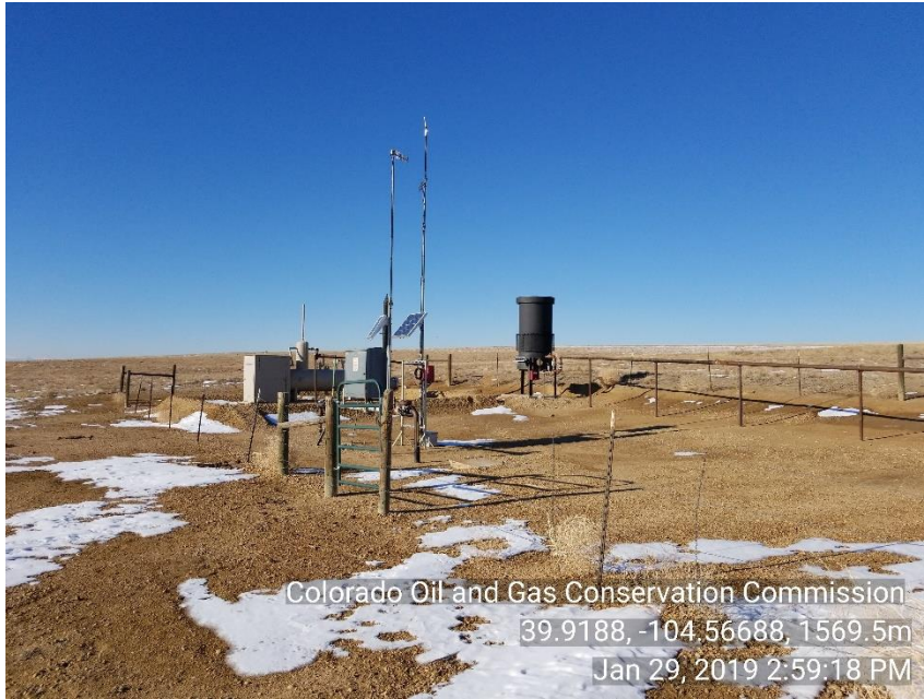
Photo 5 ECD, sep and meter run
