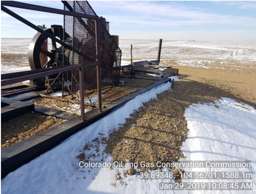
Photo 3 Stained soil removed
