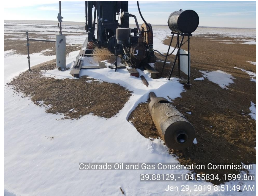
Photo 2 stained soil removed well SI
