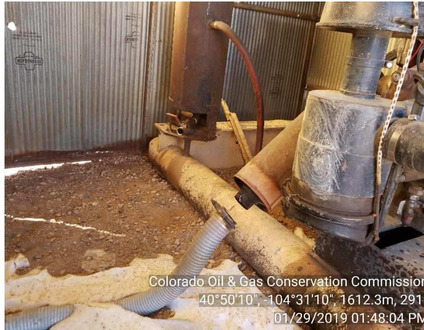
Photo 3: Tubing not fastened
