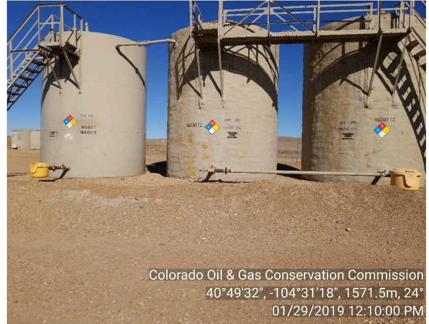
Photo 2: Tank Battery. Pictured to left, tank does not have correct labeling.
