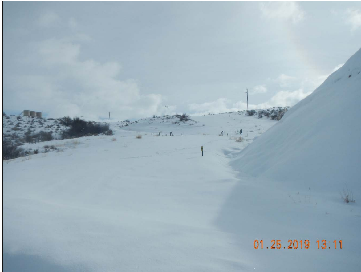
Photo 1. Overview of unmaintained access road from county road.
