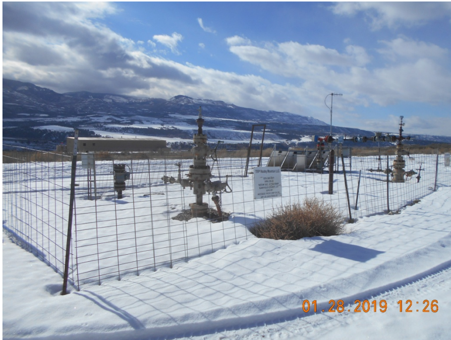
05-045-07465 Clough #RMV 215-21 wellhead
