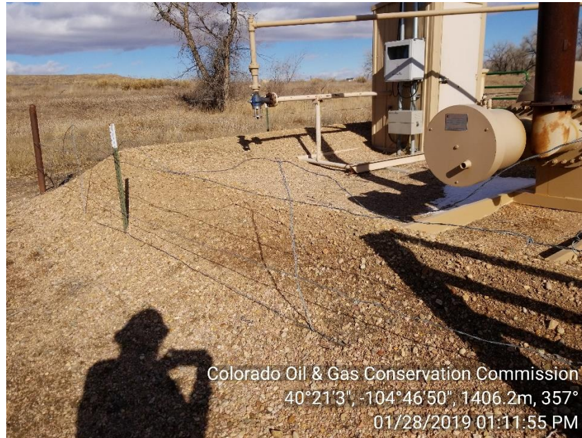
Photo 3: Fencing in disrepair around separator.
