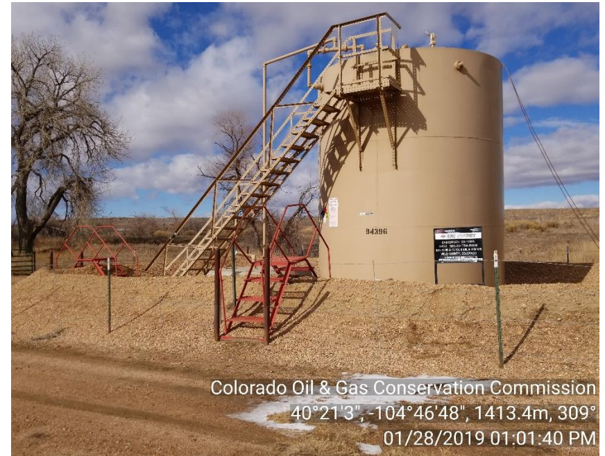
Photo 2: Tank Battery; inadequate berm (located in floodplains)
