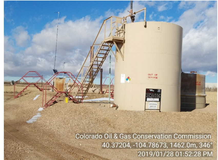
Photo #2 Coltrane-Igo # 1, Igo 28-3H6 Battery Shut-down Contents / Capacity not posted on crude oil tank
