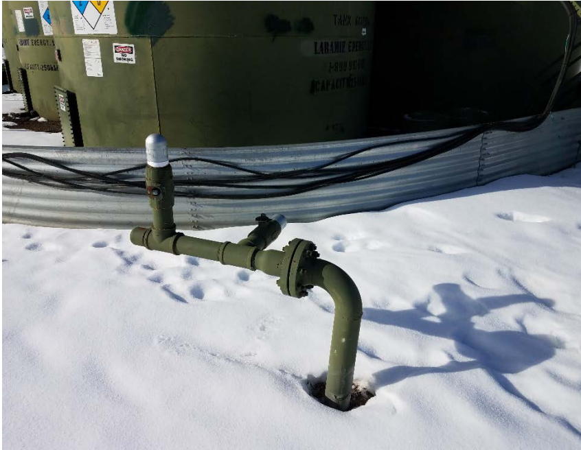
Location Photo #3, Unmarked, unused flowline riser.
