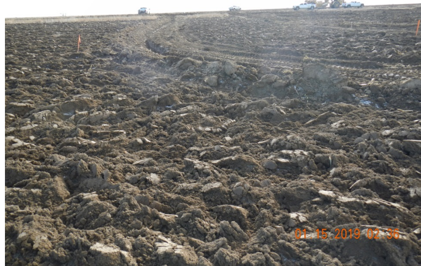
Photo 4. Photo taken from the northeastern perimeter of the location, facing South. Photo illustrates the ditch and berm BMP that has been installed around the perimeter of the location.
