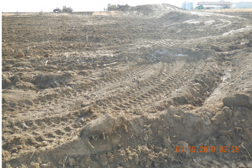
Photo 5. Photo taken from the northern perimeter of the location, facing West. Photo illustrates the topsoil salvage operations underway and has been temporarily stabilized with equipment tracking.
