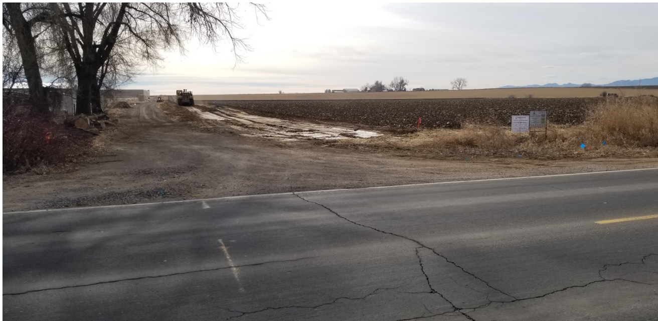
Photo 1. Photo taken from the entrance of the location off CR 20.5, facing South. Operator has started topsoil salvage operations along the access road. At the time of this inspection, no stormwater erosion issues were observed at location or along the access road.
