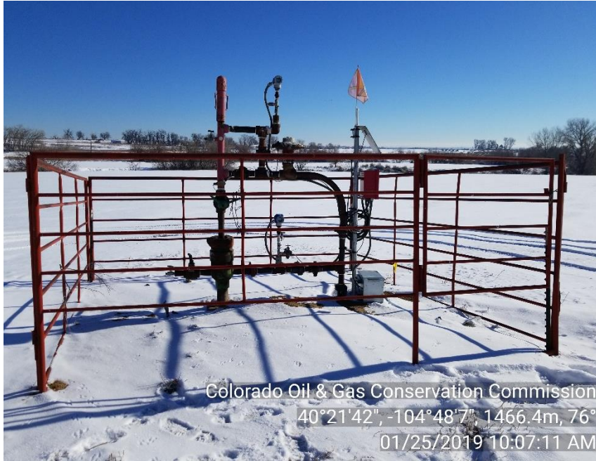
Photo 1: Wellhead with no location sign
