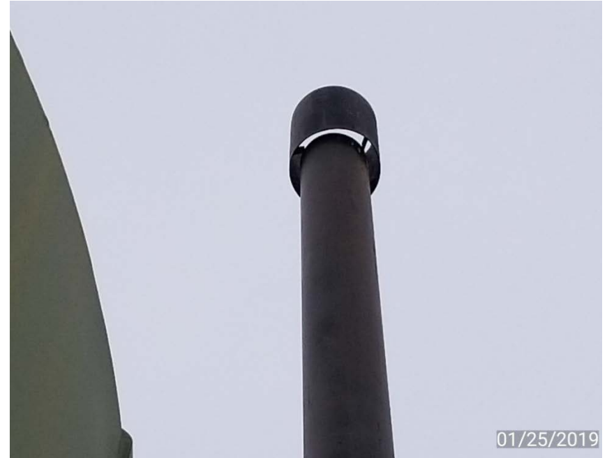
Photo 2. Bird protection not visible on oil tank stack.
