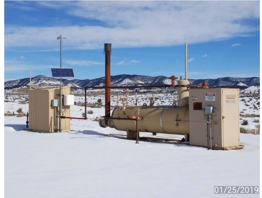
Photo 2. Meter building and separator.
