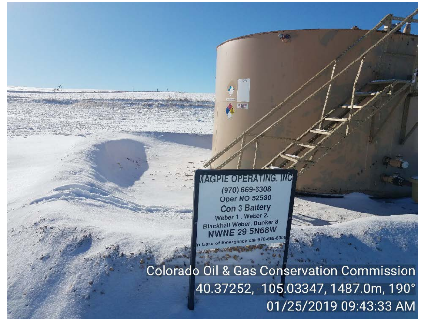
Battery sign on 1/25/19
