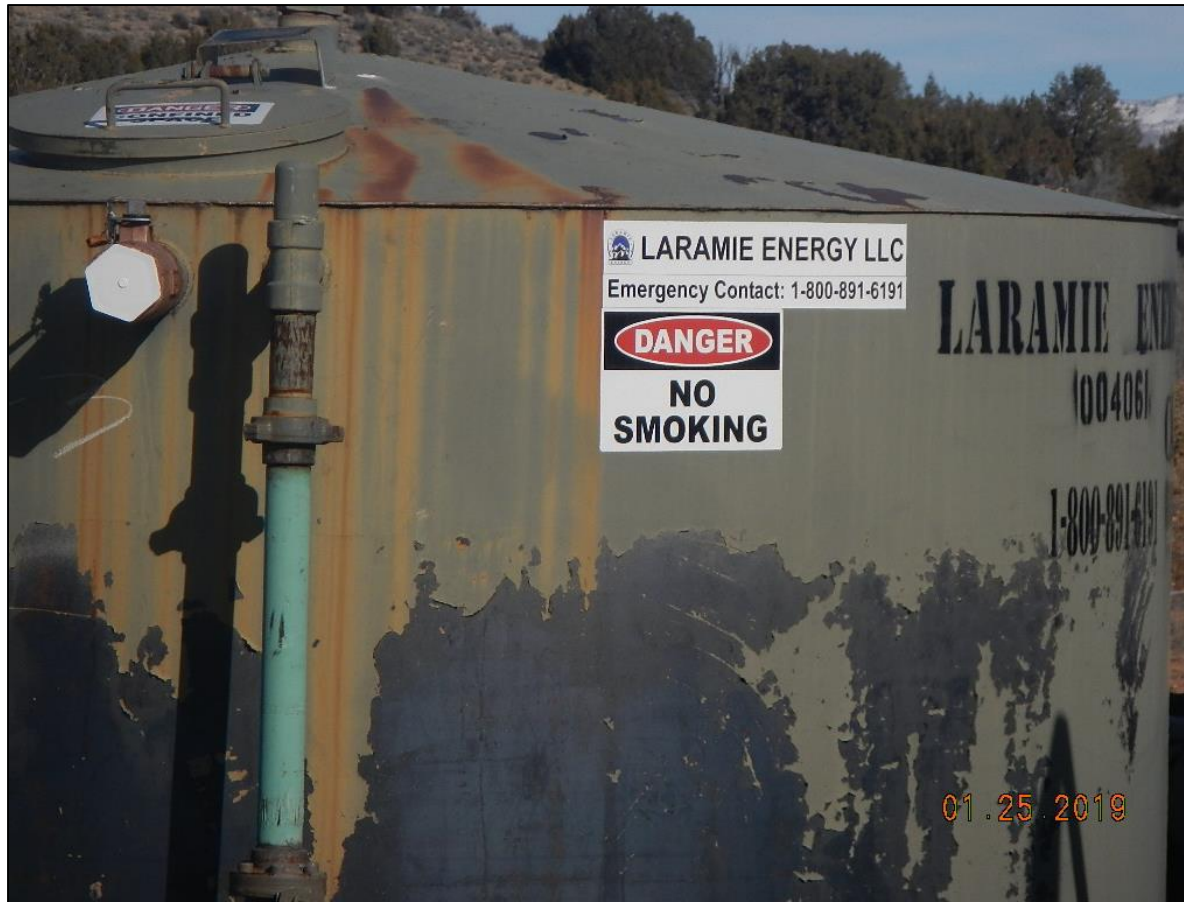
Tank battery no 911 posted on location
