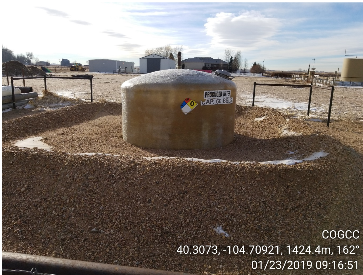
Photo 5 – Produced water vault on location
