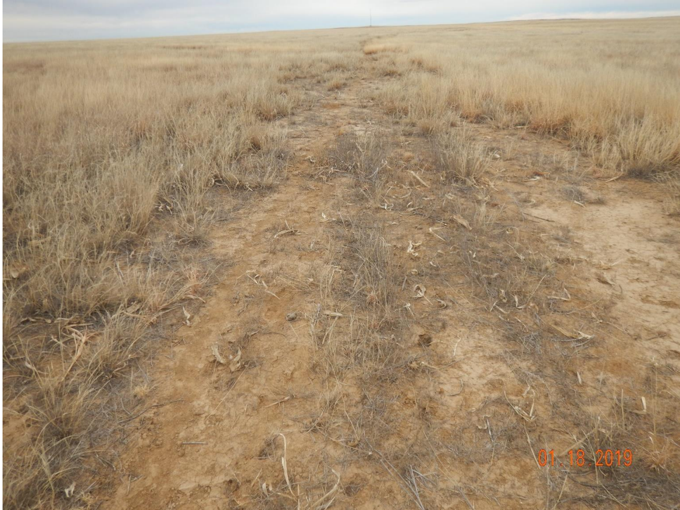
Photo 14: Photo taken from the north end of the location, facing north. Photo shows access road. Though there are areas of the access road where vegetation establishment is occurring, vegetation establishment is not uniform; access road remains predominantly bare and exposed soil.
