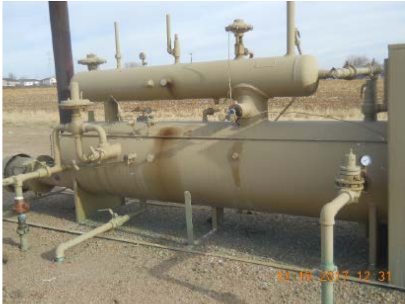
Photo #6 Strong 4-22 Separator Leaking fittings from prev. FIR
