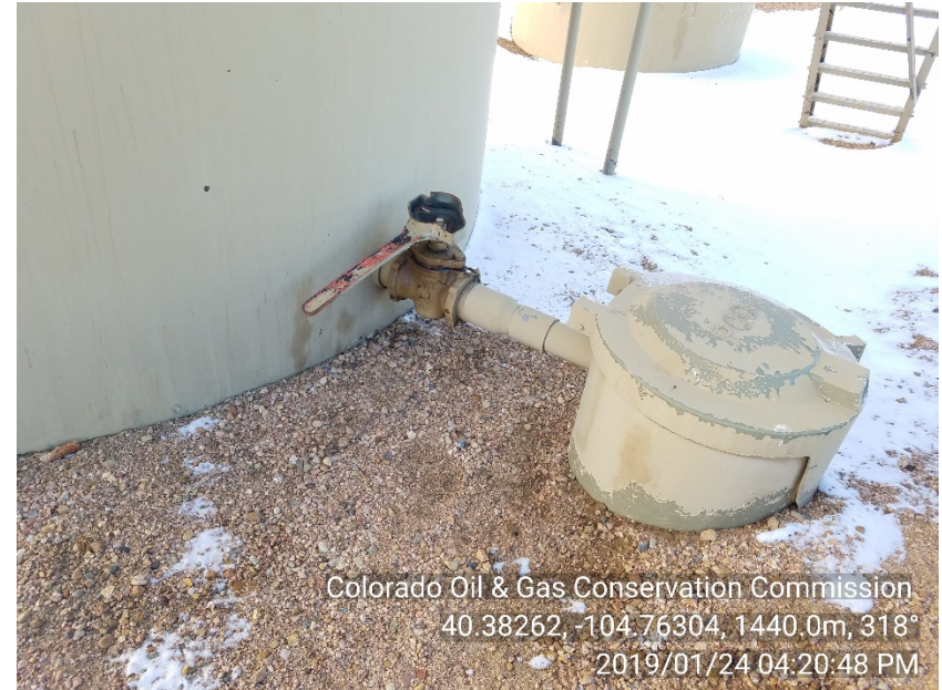
Photo #5 Strong 4-22 Oil Tank Stained soil under Loadout Appears mitigated
