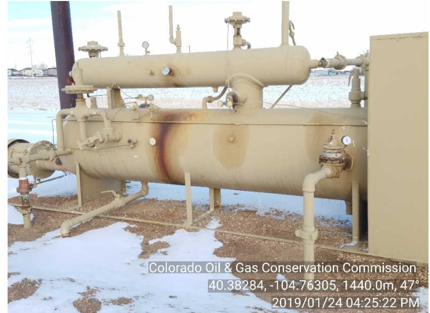
Photo #7 Strong 4-22 Oil Tank Leaking fittings Appears mitigated Stains are dry. No soil stains
