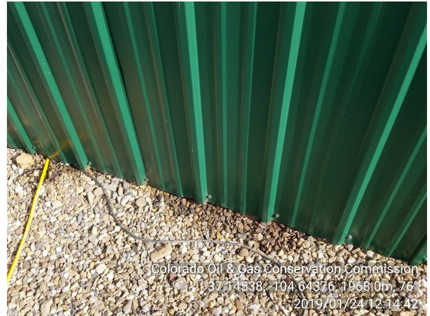
PHOTO 6: STAINED SOIL SPREADING UNDER SOUND WALL ON WEST SIDE.
