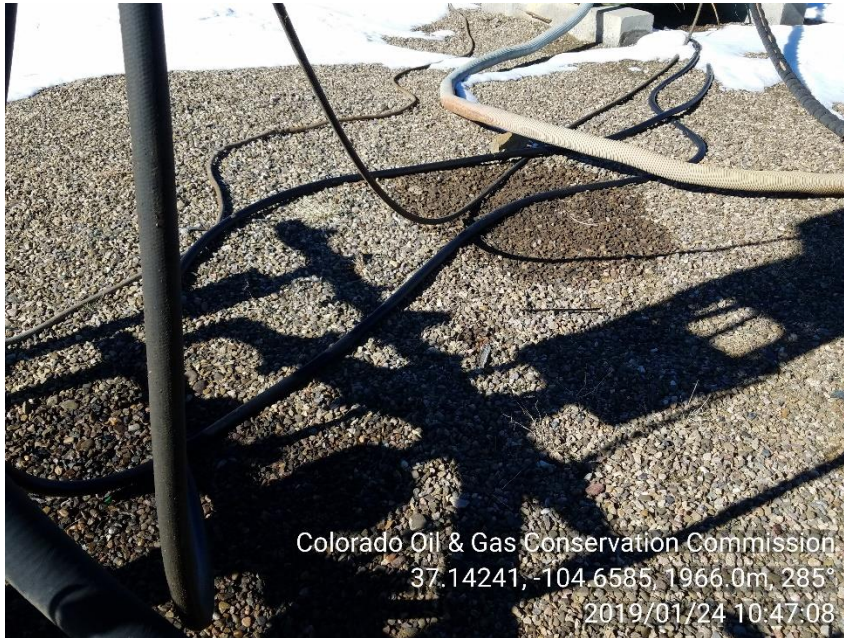
PHOTO 3: STAINED SOIL AROUND WELLHEAD AND BETWEEN ENGINE SKID.
