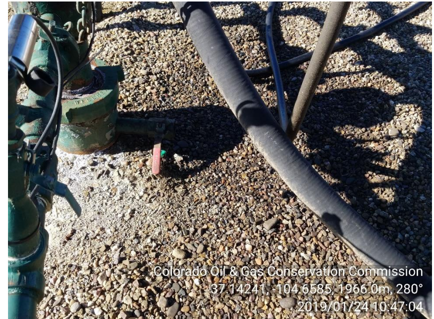
PHOTO 4: STAINED SOIL NEAR WELLHEAD
