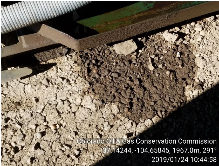
PHOTO 3: STAINED SOIL UNDER DRAIN PLUG ON COMPRESSOR SKED.
