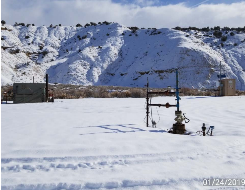
Photo 3. Well head, separator, and gas meter run.
