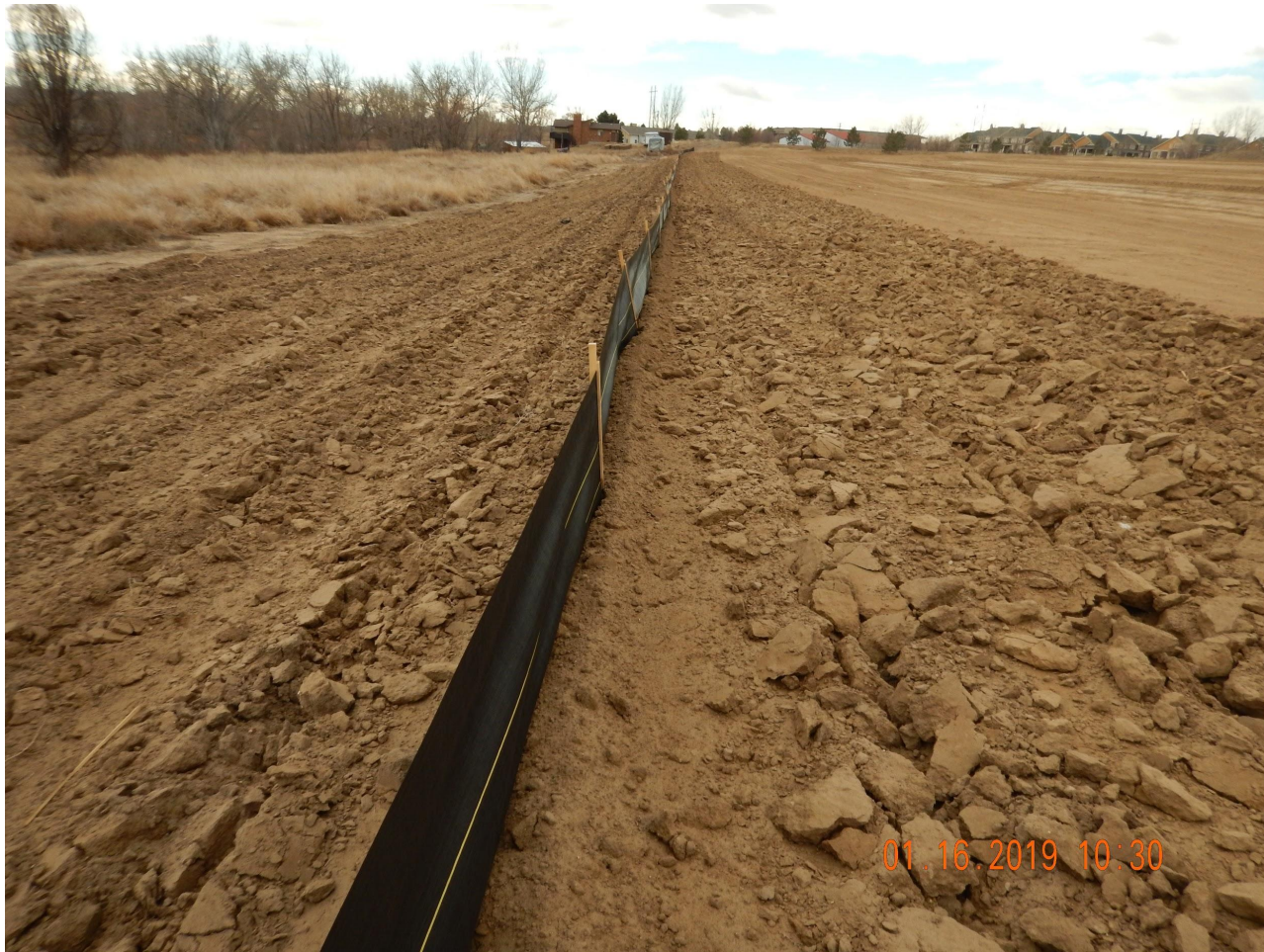
Photo 1. Photo taken from the northeastern perimeter of location, facing South. Final reclamation is in-process. Surface roughening and silt fence BMP have been implemented along the toe of the disturbance area.
