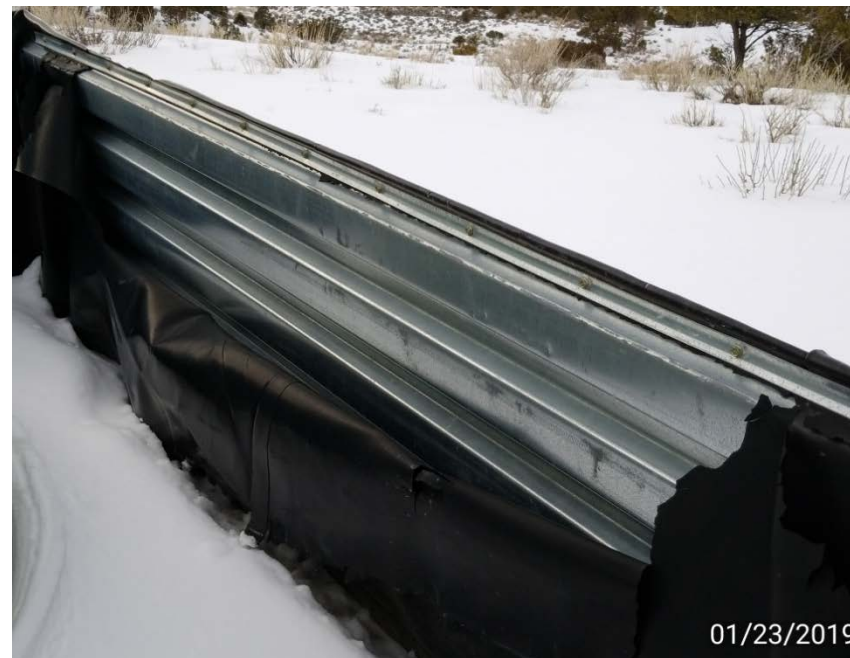
Photo 2. Secondary containment liner for tank is torn .
